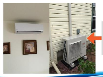
A ductless mini split system will have the required information on the outside unit. Only the unit make, model, and serial number is needed as the compressor is not accessible.
