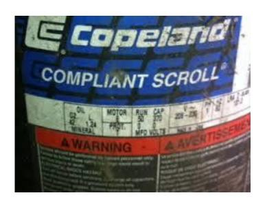
Typically, the compressor oil charge will be stamped on the compressor label.
